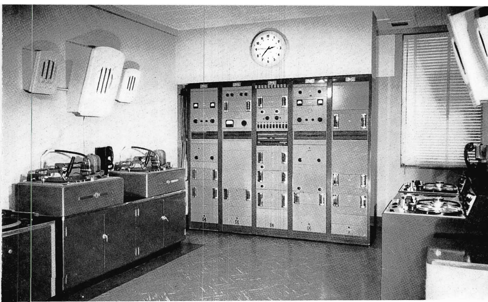
FIG. 31. WBAP's recording room is one of the finest station recording setups in existence. At left, in the view above, are the RCA 73-B Professional Disc Recorders. At right are two studio-type tape recorders. Racks in the center house line amplifiers, recording amplifiers, monitoring amplifiers, power supplies, switching facilities and the auxiliary equipment.
