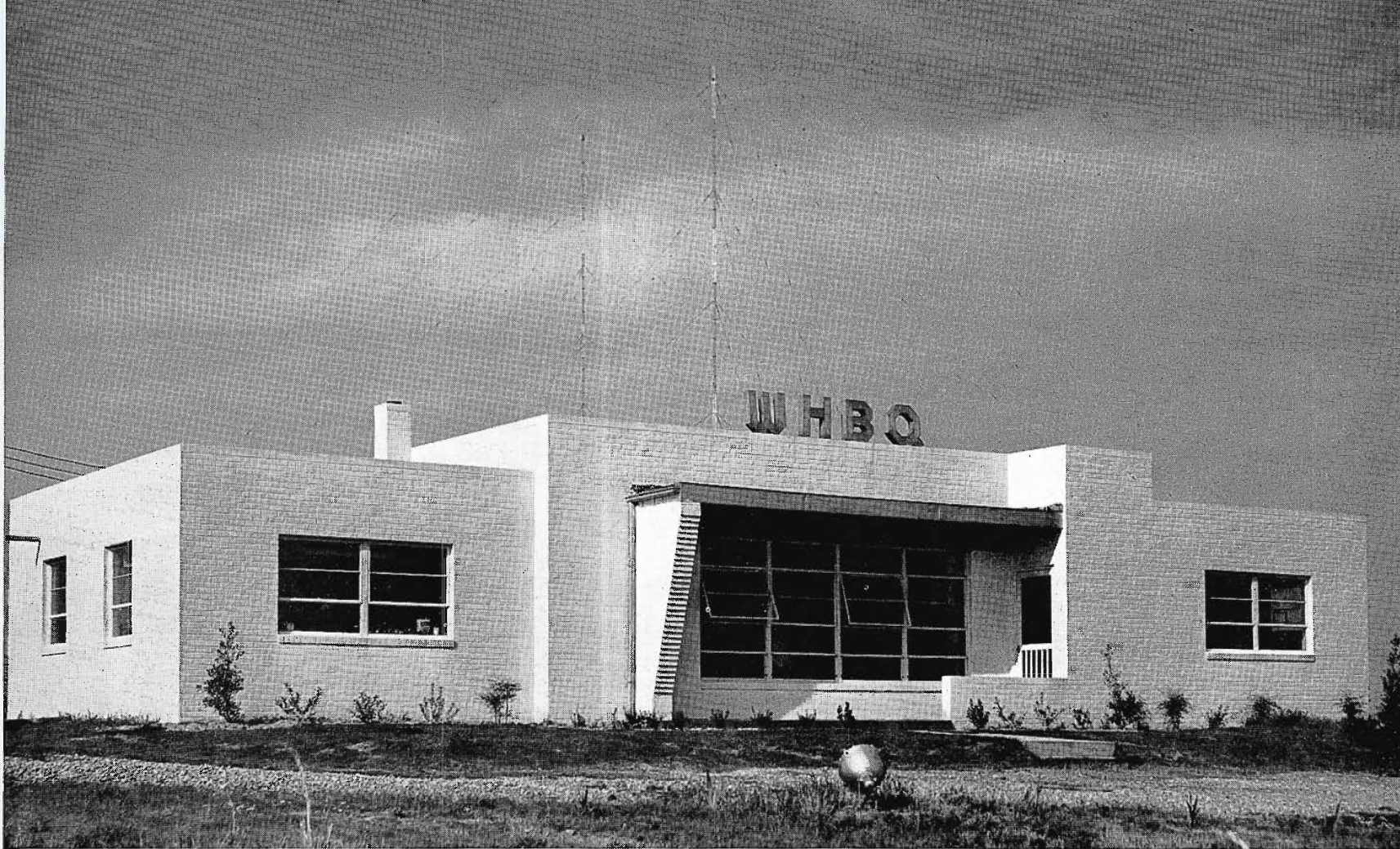
FIG. 1. The WHBQ 5000-watt transmitter building, with its solar-type front facing south. Two of the five 315-foot towers are visible in the background.
