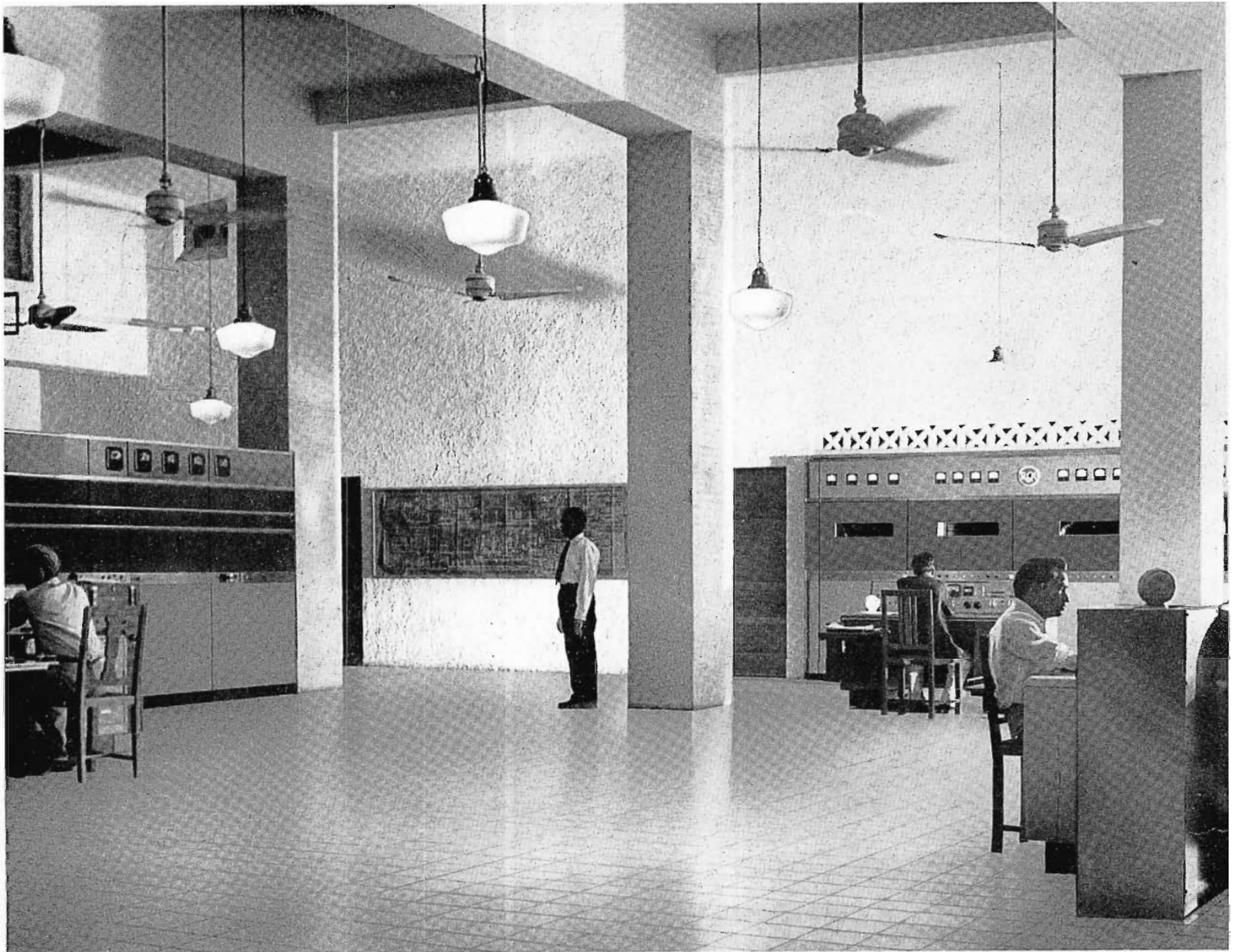
The spacious Transmitter Hall is equipped with two RCA 50 kilowatt, dual-channel, high frequency broadcast transmitters and one RCA 10 kilowatt medium frequency broadcast transmitter. The building has been designed so that additional equipment may be installed and additional construction carried out for future expansion.
