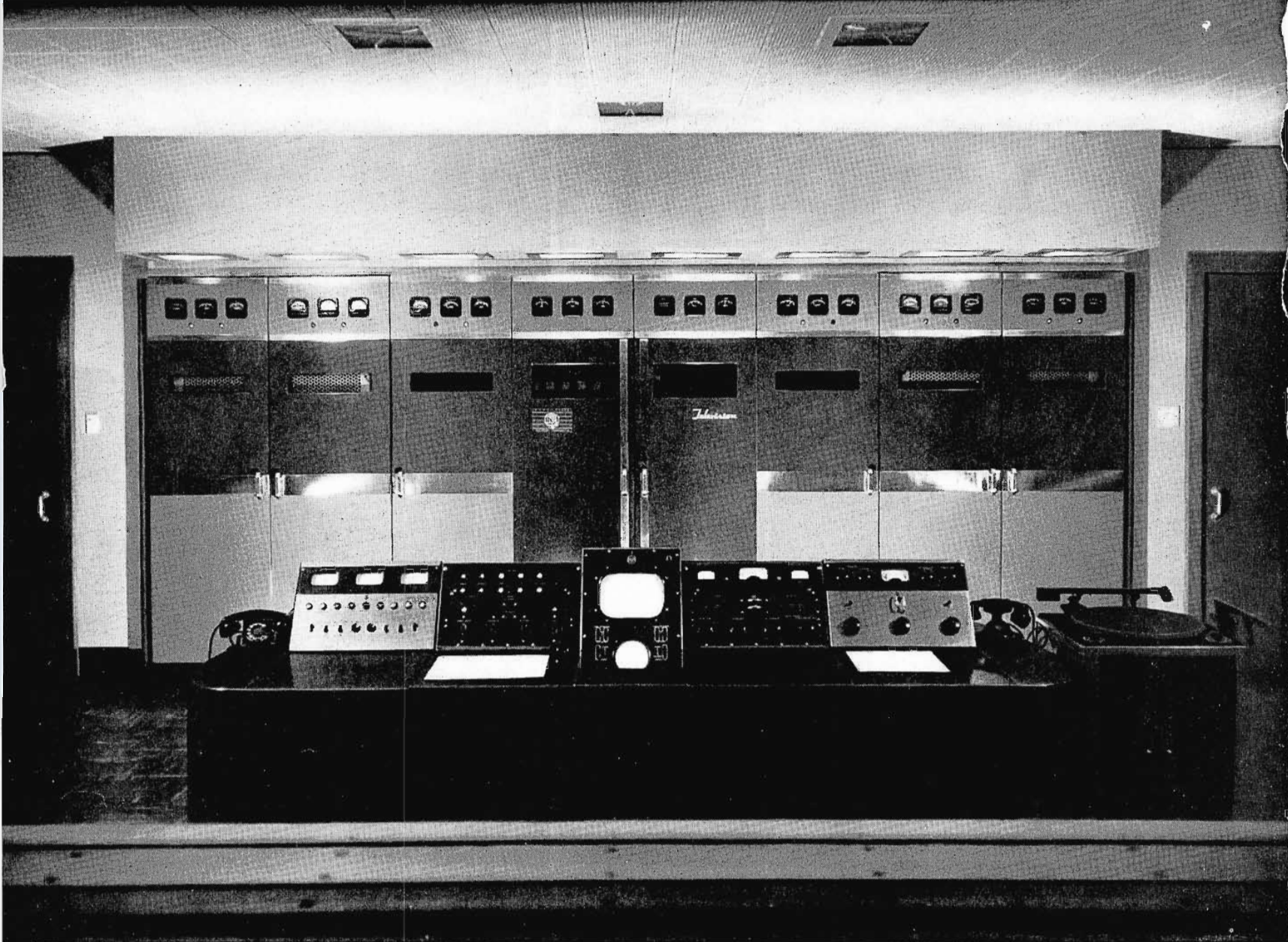
FIG. 17. WBAP's RCA TT-5A Television Transmitter as seen through the window from the corridor which runs the length of the TV area of the building. The control console contains the operating controls for both the TV and the FM transmitters.
