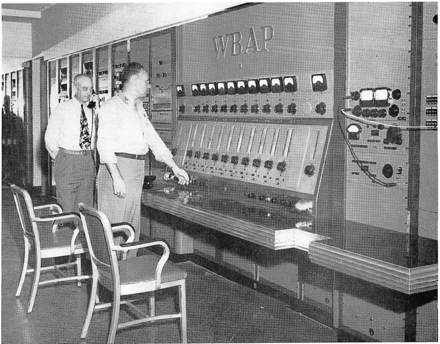
FIG. 3. This is a closeup of the main operating position of the WBAP master control position. The special four-rack-wide control section was custom-built by RCA to WBAP's specifications. It provides means of switching sixteen incoming circuits to any or several of ten outgoing circuits with complete "preset" facilities. Arrangement of controls is shown in diagram, Fig. 4, on opposite page. Operation is described in the text. Shown in this view are, at left, R. C. Stinson, Technical Director of WBAP, under whose direction this equipment was planned and installed; and, at right, Roy Bond, of the WBAP engineering staff.
