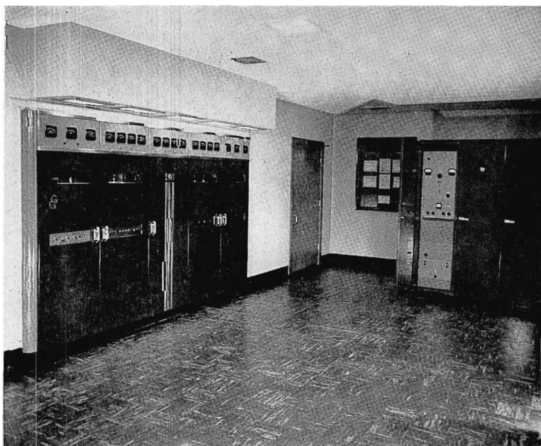
FIG. 20 (below). Looking toward the FM end of the transmitter room. The three cabinet racks at the far end contain the audio input and monitoring amplifiers, monitors and test equipment.
