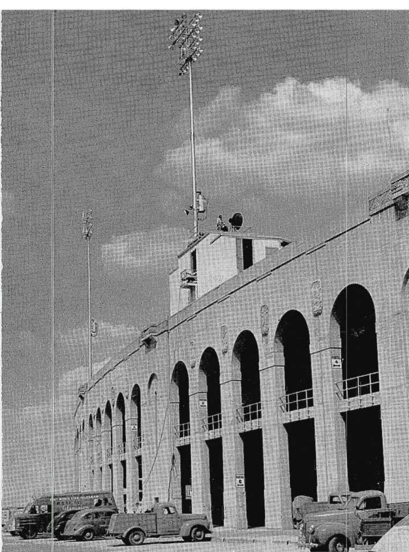
FIG. 23. For pickups at the stadium, ball park and similar events, WBAP leaves the control equipment in the mobile unit, uses long cables to cameras and microwave parabola located at vantage points.
