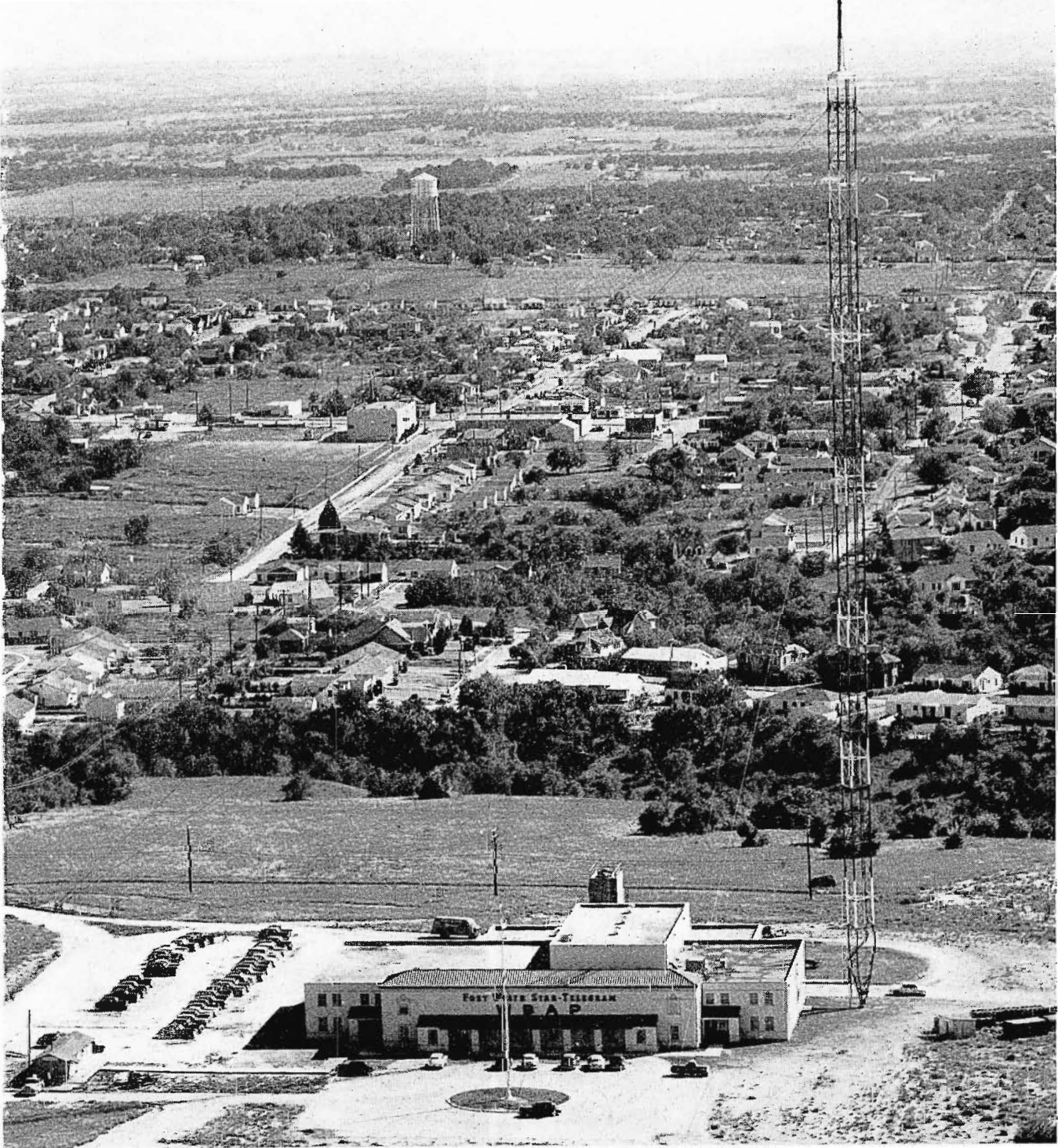
FIG. 3. Front of the WBAP building from the air. The antenna tower is 25 feet from the building and is located immediately adjacent to the transmitter room so that transmission lines are as short as possible.
